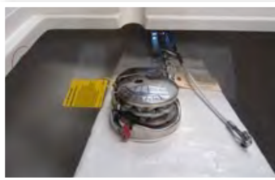
Windlass anchor roller, as seen from the anchor locker
