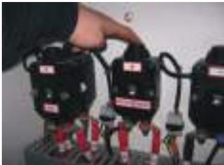
Electrical battery switches 12V -
