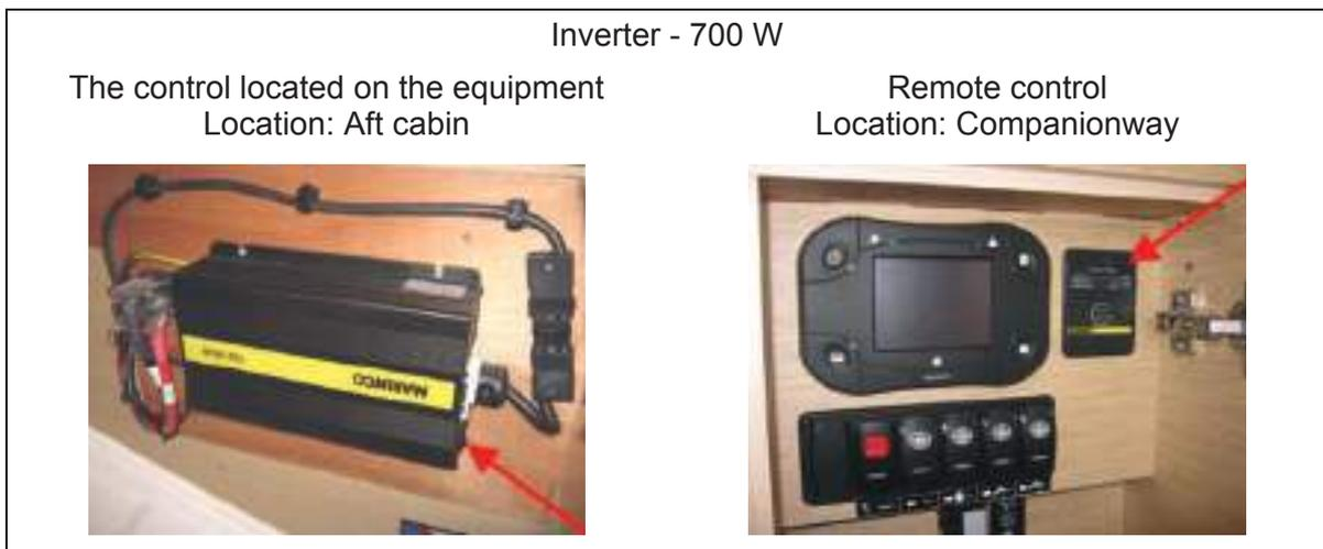
The power to the inverter must only be supplied by lead batteries.
