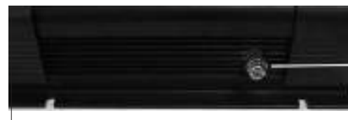
DC Grounding Connection (DC Case / Chassis Ground ⚡) see system wiring illustrations on page 11
