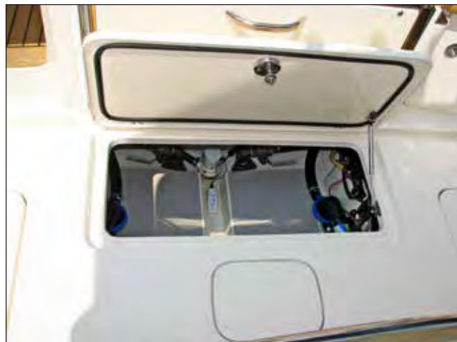
Aft Under Deck Systems Compartment
