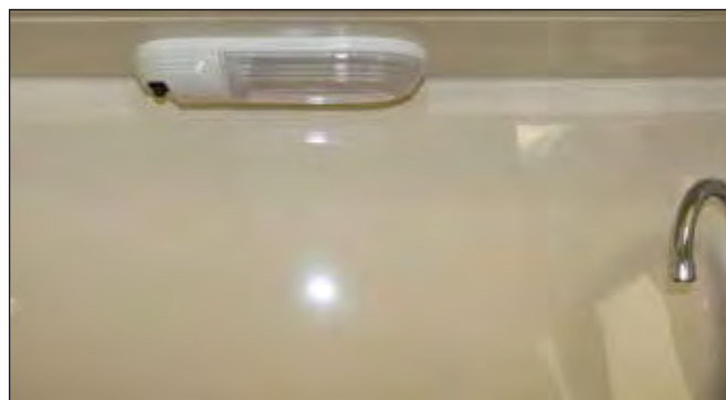
Sink Overhead Light & Switch
