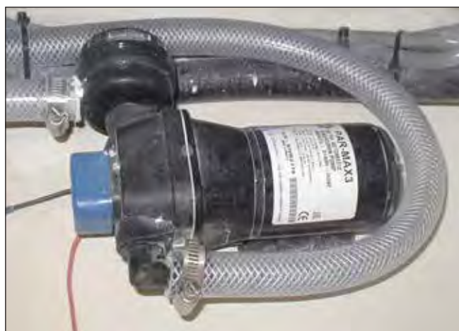
Typical Fresh Water Pump & Strainer
