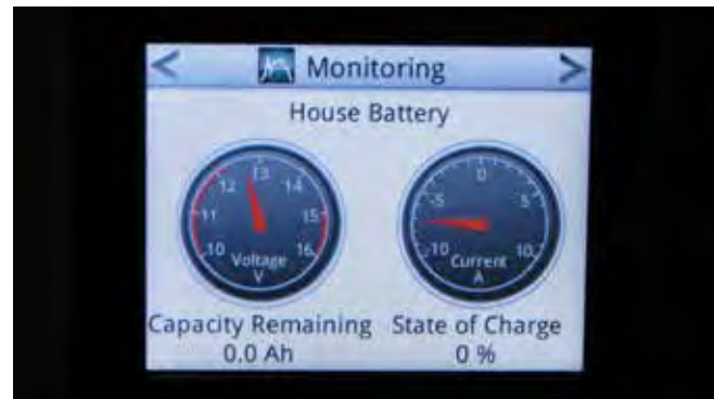
DC Power Meter
