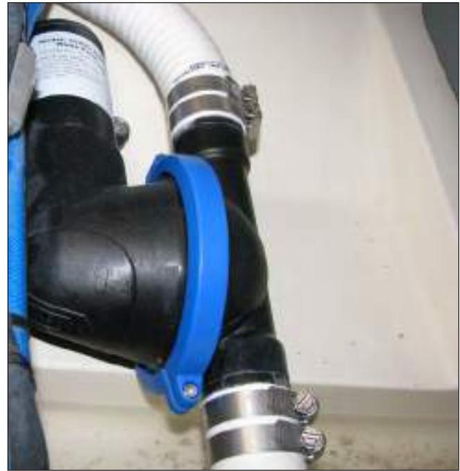
Typical Waste Discharge Diaphragm Pump
