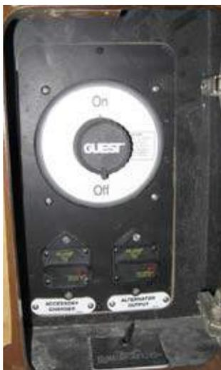
Electricity from the battery to the Safety Breaker Panel is controlled by a master disconnect switch. This switch is located in a cabinet in the starboard side of the salon. To provide electricity to the Safety Breaker Panel, turn the master disconnect switch to the ON position. Circuit breakers on the Safety Breaker Panel control the other DC circuit breaker panels.
