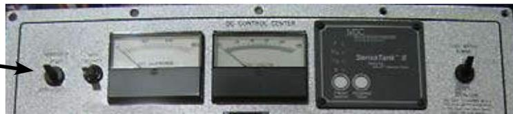
8. Push the switch to the **START** position and hold it there until the generator starts. Release the switch when the generator starts.
