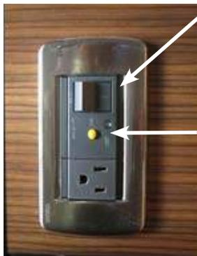
GFCIs have Test and Reset buttons located on the receptacles. To reset the GFCI after it has tripped, press the Reset button. Resetting a GFCI allows electricity to flow again to the receptacle.
