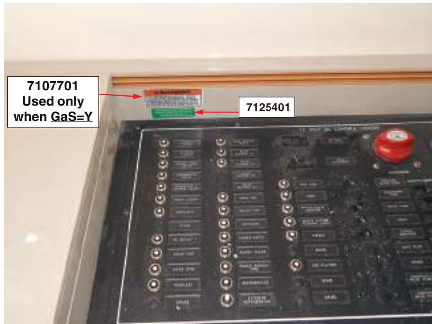
Figure 2-7 – Labels Required at 12V Panel
